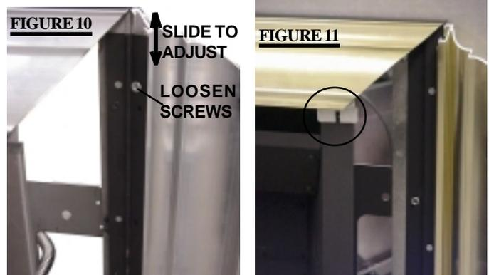
To adjust the trim: If the mitre is out of alignment, open each side and loosen the two screws at either side trim hinge. Slide the trim up or down to adjust and re-tighten screws. There is also a very slight in/out adjustment that can be made.
